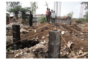
Church Basement work at Goudanahalli
